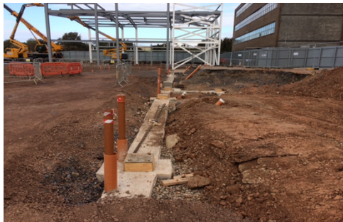
3 Ground beam foundations and drainage
