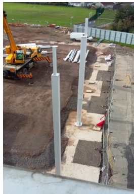
1 First Steel Columns of Sports Hall erected
