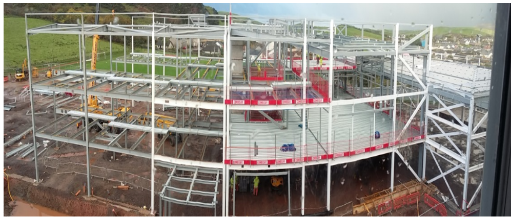
12 and 13 Panoramic views of new school building
