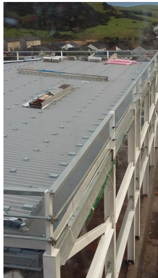
10 Progress on Sports Hall Roof
