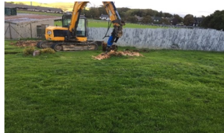
15 Tree stumps cored out at the current bus drop-off area
