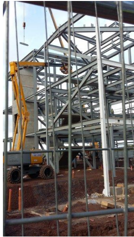
8 Complexity of the steelwork
