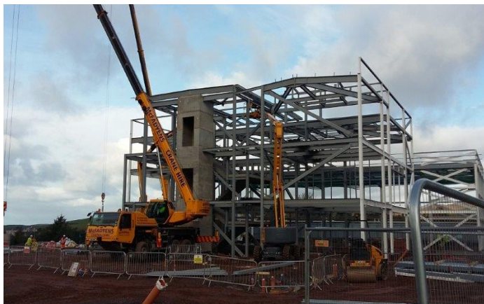
5 Steel frame and lift shaft No. 1
