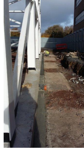
7 Foundations for erection of the blockwork in place
