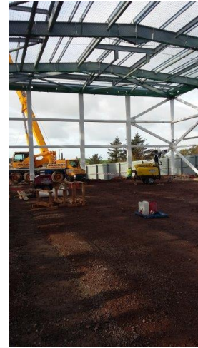
9 Roofing works commence on Sports Hall
