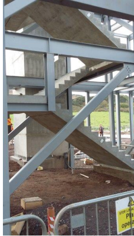
6 Staircase No. 1 installed
