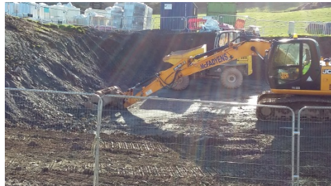
14 Reducing levels for 3G pitch installation in Phase 2
