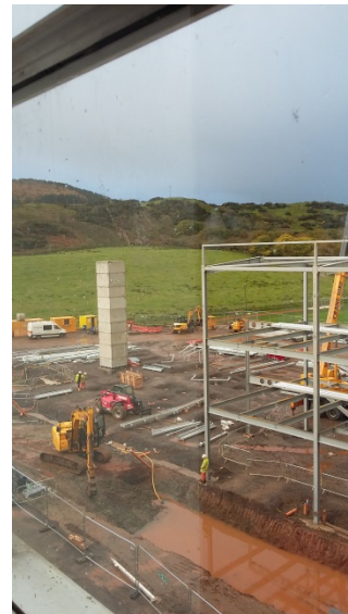
11 Building edging towards lift shaft No.2
